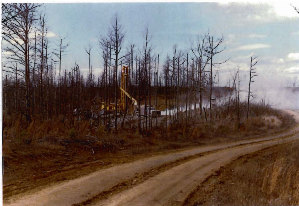
Figure 20. Drilling activity within 100 feet (30m) of the projected lineament in Example 7.
