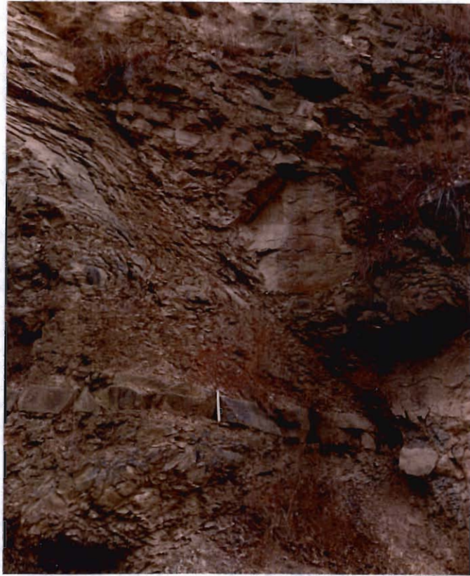
Figure 15. Closer view of one of the fractures at Field Station 55. The scale equals one foot (30.48cm).
